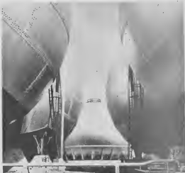
A NEAR perfect balanced composition of spheres plainly shows their lap-riveted construction and supports. UN COMPOSICION casi perfectamente balancea di tanki rondó claramente ta muntra nan construcion y aguanje geweldo.
